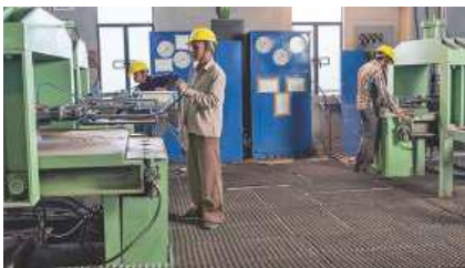
Valve testing area.
