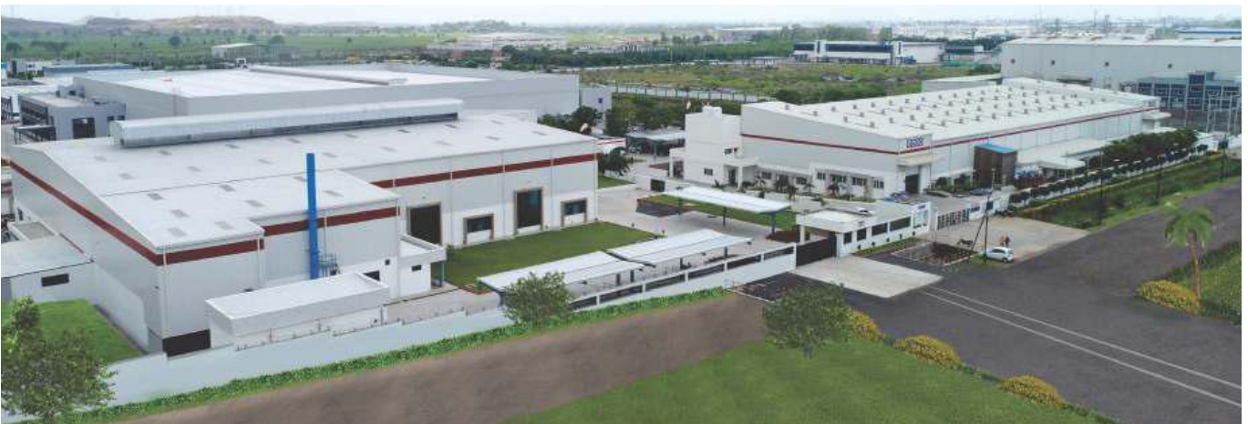
Unit 3 & 4, SEZ, Pithampur with built up area spanning over 100,000 Sq. feet
