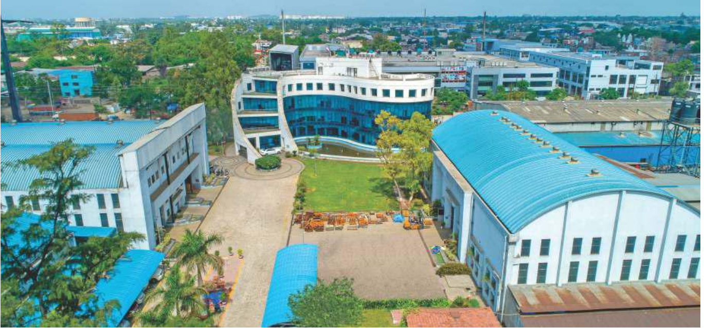
Unit 1, Indore with built up area spanning over 125,000 Sq. feet
