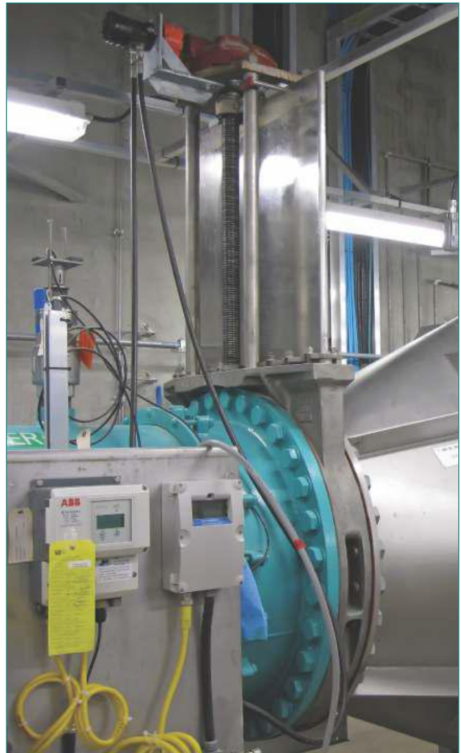
DN 1500 (60") valve as supplied to Yukon Energy Corporation, Canada.
