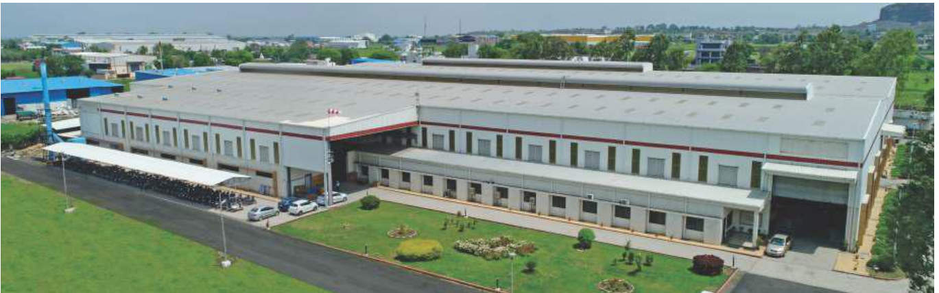
Unit 2, Indore with built up area spanning over 155,000 Sq. feet
