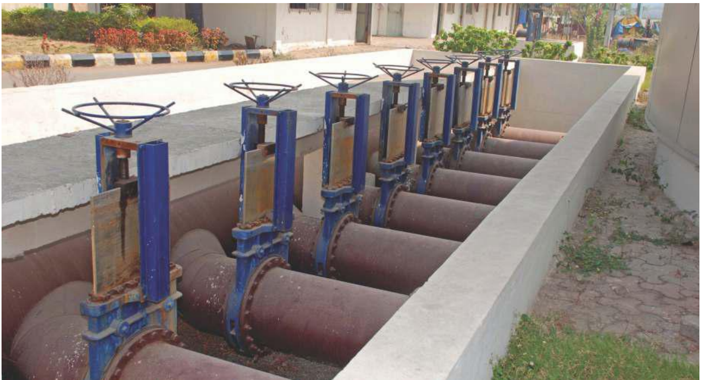
Installation of unidirectional DN 600 (24"), supplied for Sewage treatment plant, Nerul, Mumbai
