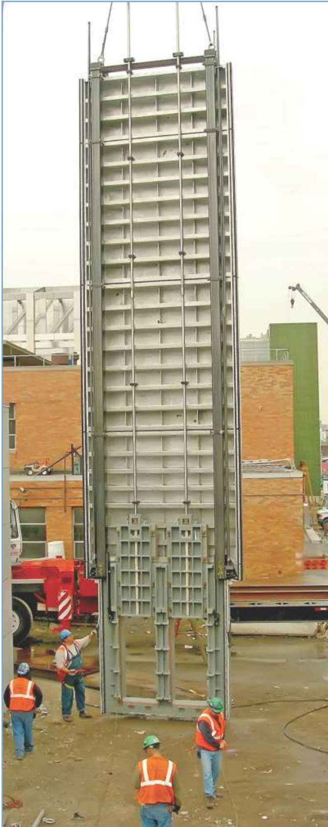
3200 x 13420 mm Bulkhead Gate with Integral Slide Gate for Newtown Creek, NY, USA
