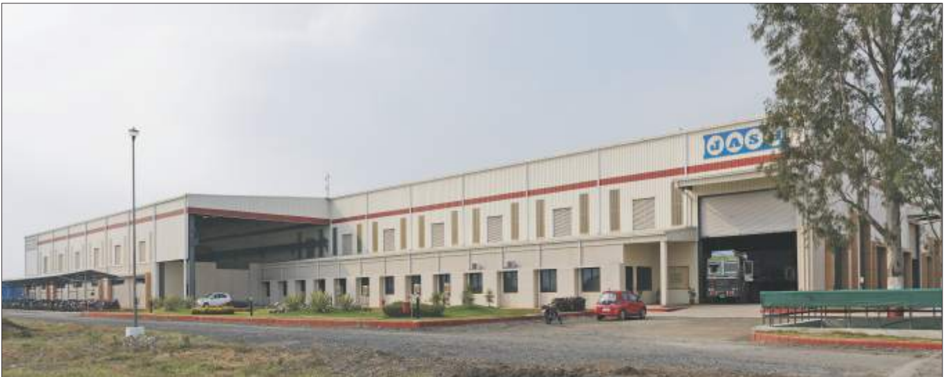
Unit 2: Fabricated Products Plant, Bardari, Indore
