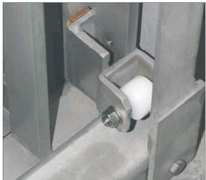
Guide Roller Arrangement
