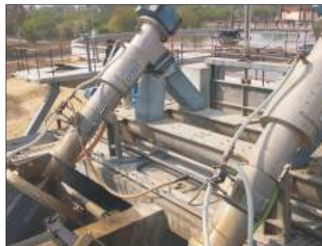
Rotary Drum Screen for STP New Delhi, India
