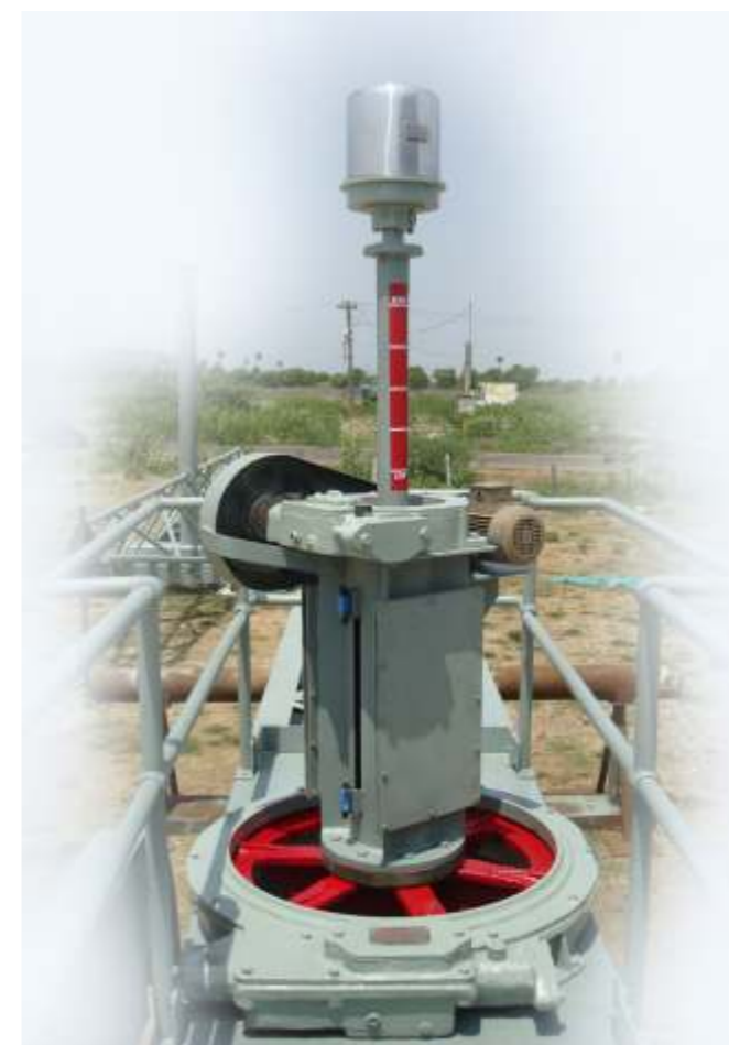
Motorized lifting device with slip ring assembly
