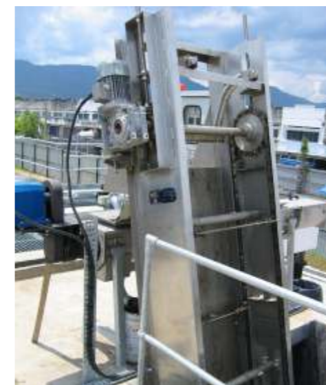
Type SP-M2-C Mechanical Fine Screen Taman Mas, Sewage Treatment Plant, Malaysia
