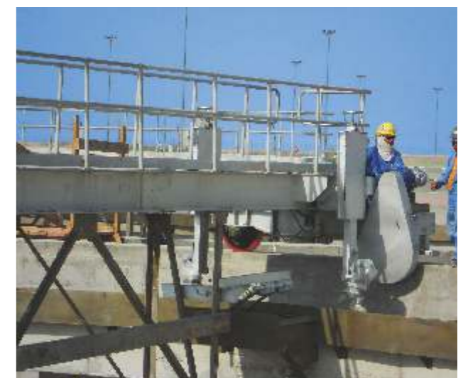
Type SPC-B Peripheral driven Traction Clarifier drive assembly, Skimmer Assembly and Weir cleaning device – Doha STP, Qatar
