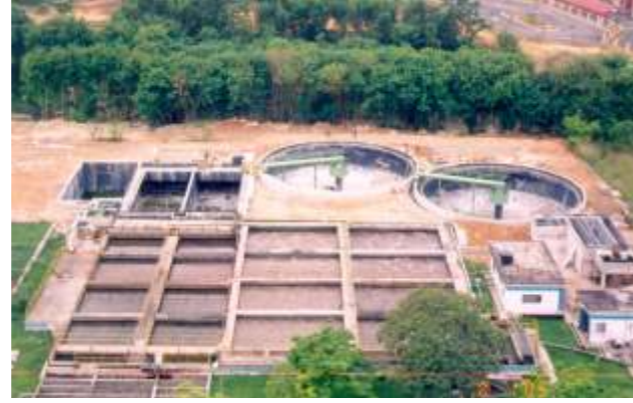
STP at Damansara, West Malaysia
