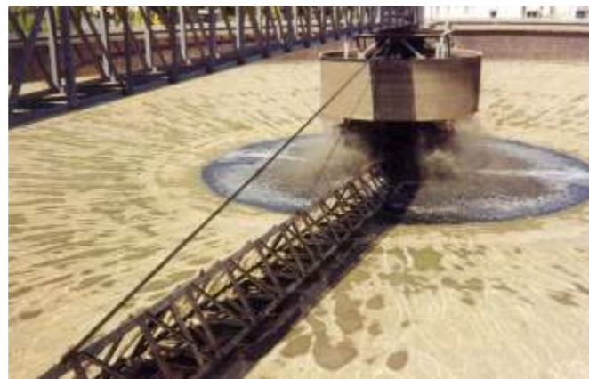
Type SPC-C: Centre Pier Type Clarifier
