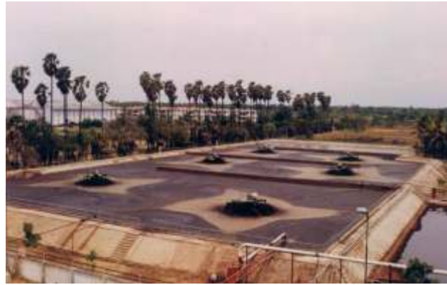
Distillery ETP at Thiru Arooran Sugars, Tamilnadu
