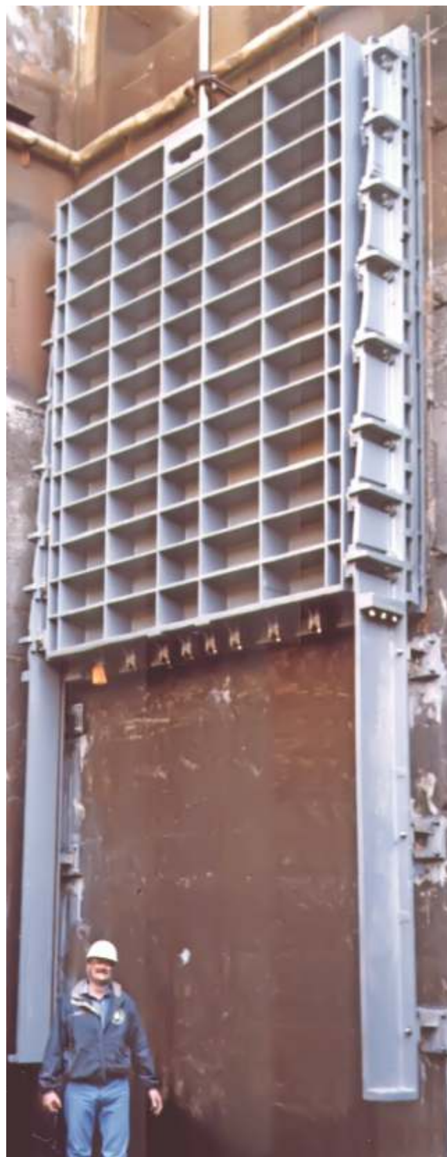
3350 x 3960 mm Inverted Cast Iron Slide Gates at Vermont Yankee Vernon, VT, USA
