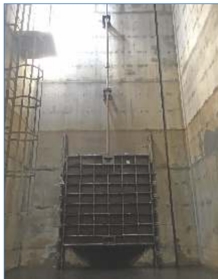
3000 x 3000 mm Cast Iron Slide Gates at Langat-2 WTP & WRS, Kuala Lumpur, Malaysia
