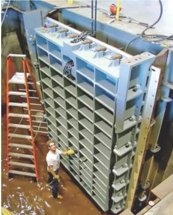
2750 x 3800 mm Cast Iron Glydaseal™ Slide Gates for Paerdegat Basin Brooklyn, NY, USA
