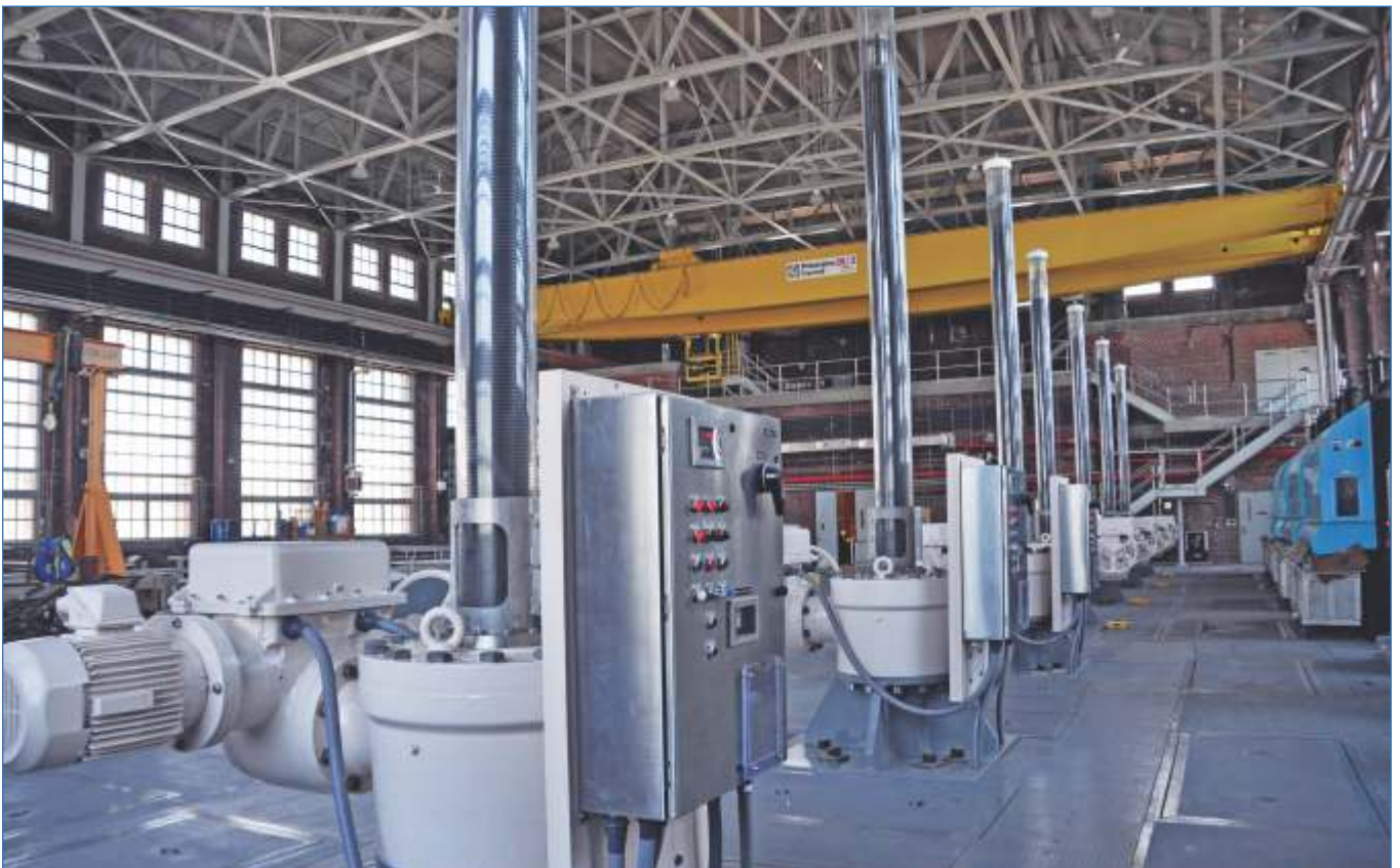
1800 x 3000 mm Cast Iron Slide Gates at NYC DEP's West Branch Res. Carmel, NY, USA
