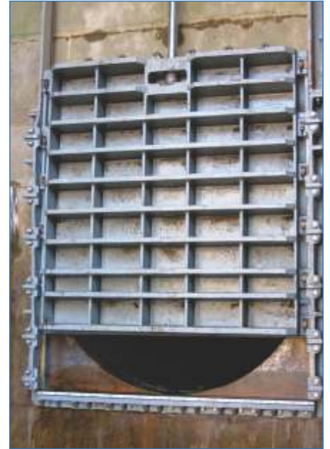
2700 x 2700 mm Cast Iron Slide Gates at Woodward Dam, Oakdale, CA, USA
