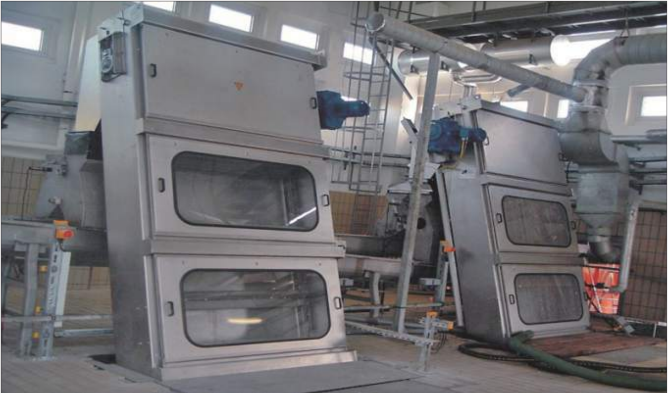
“MM2MM”™ Multirake Screen with Top Enclosure
